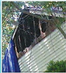
Exterior walls with holes, breaks or loose and rotting materials
