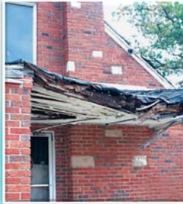
Exterior walls with holes, breaks or loose and rotting materials
