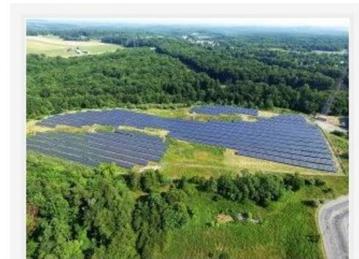
Maryland, site of the Montgomery County microgrid project, pictured, is funding 14 new projects. Photo courtesy of Schneider Electric
