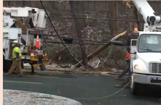
Figure 14. Downed powerlines resulting from the ice storm (WUSA9).
