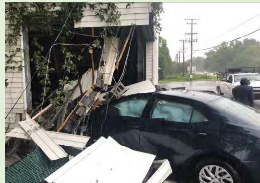
Figure 25. Property damage resulting from Tropical Storm Isaias. ( Prince George's County Fire/EMS Department Twitter ).
