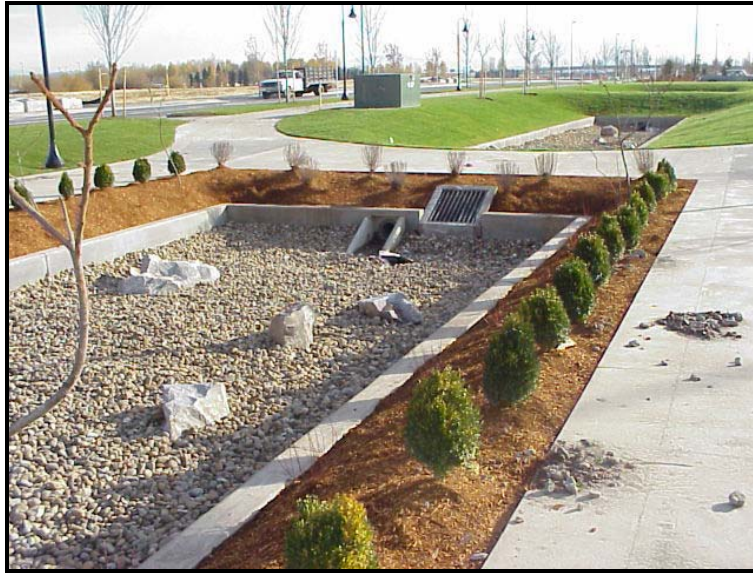
Figure 10 Sand Filters (Source: East Baton Rouge Parish-Stormwater BMPs)
