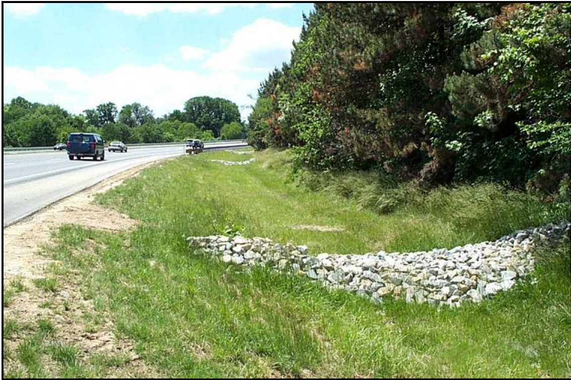
Figure 44 Check Dam (Source: NPDES, DOT, New castle County, Delaware)
