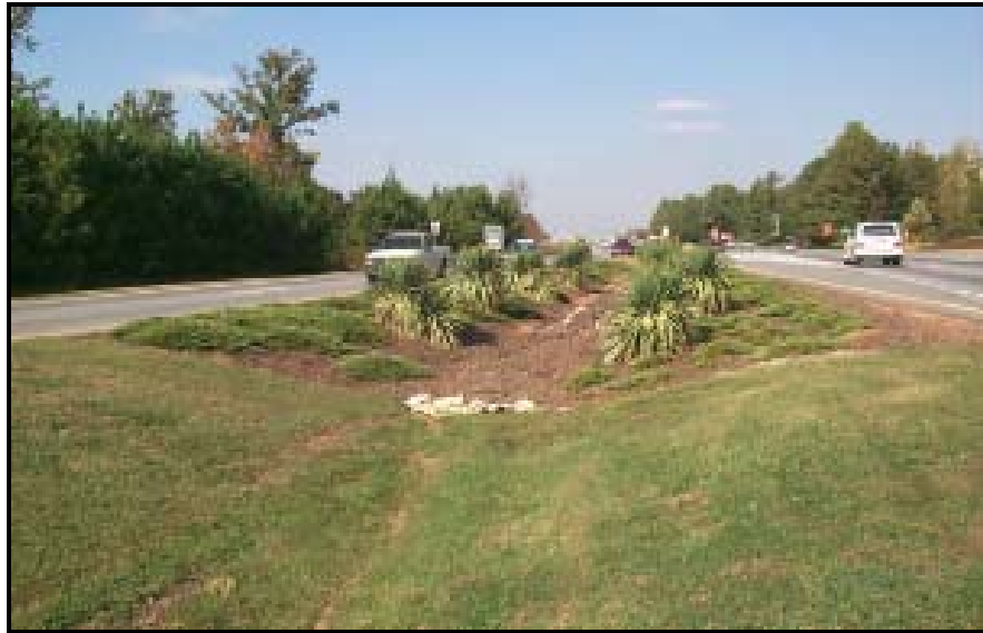
Figure 2 Dry Swale
