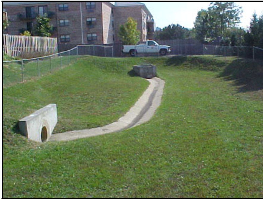
Figure 32 Dry Pond (Source: Fairfax County, VA)
