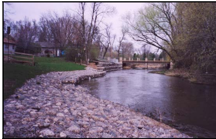
Figure 46 Gabion (Source: Best Management Practices, redwood-Cottonwood River Control Area (RCRCA))
